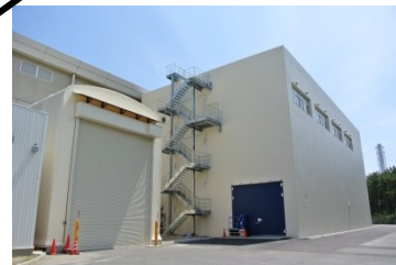
COMET & Control room
