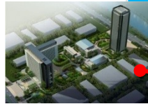
R&D Center of Heavy Ion Applications, New Campus in Lanzhou
